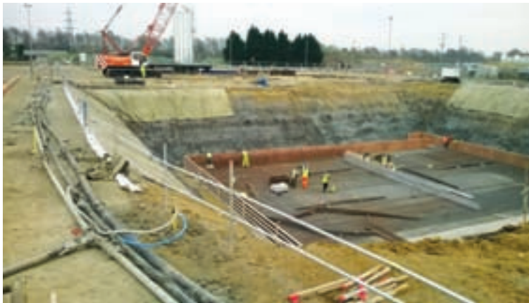
Dewatering applications: a cofferdam (above); inside a factory (above right); and an excavation (right)
