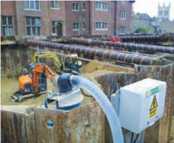
Dewatering applications: a cofferdam (above); inside a factory (above right); and an excavation (right)
