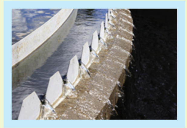
Figure 4. Clarifier weir overflow with scum baffle.
