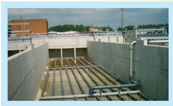
Figure 2. Diffused aeration system
