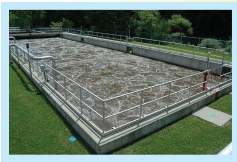
Figure 1. Activated sludge aeration basin with submerged aeration.
