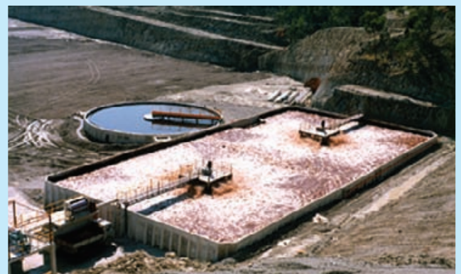
Figure 3. Fixed mounted surface aerators with a clarifier
