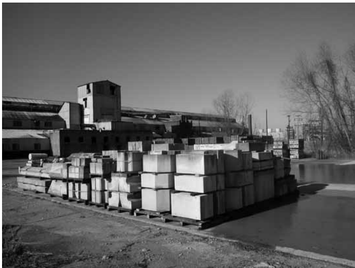
Figure 1: The complete limestone front elevation of the Wagoner Mortuary Building, stacked, sorted, labeled and recorded. Photograph courtesy of Michael Allen.
