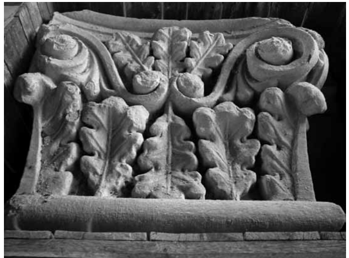
Figure 3: Marble pilaster capital from the Century Building, demolished amid national controversy in 2006. Photograph courtesy of Michael Allen.
