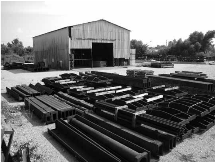
Figure 4: Part of the Foundation's collection of over 120 cast iron storefront systems, originally produced by Mesker Steel Company and other leading firms. Photograph courtesy of Michael Allen.
