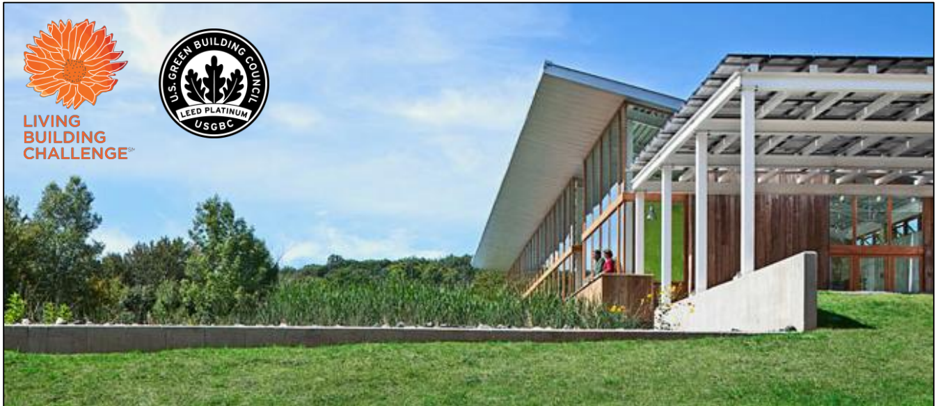
Exterior view of OCSL building and treatment wetlands
