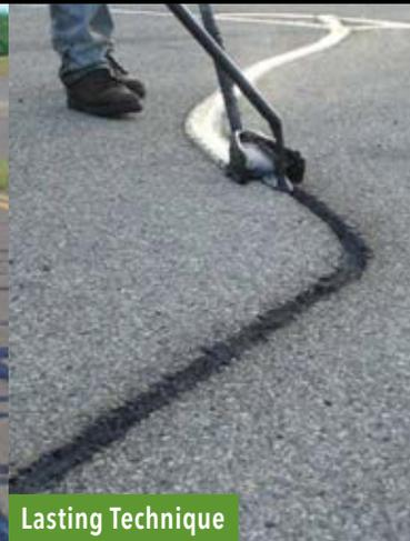
Finishing: GSB-88® penetrates down and becomes part of the surface, sealing and binding aggregates tightly together.
