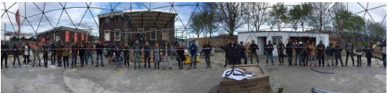
Panoramic during the construction of the geodesic dome which became the Good Chance theatre.
