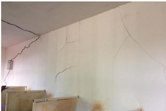
**Figure 4: Cracks in the walls of the old lab**
