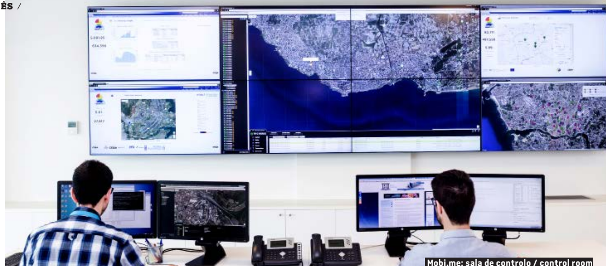
Mobi.me: sala de controlo / control room
