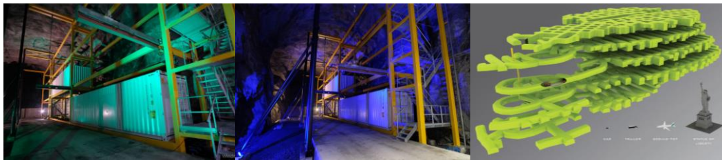
Figure 1. Underground view of Lefdal Mine Datacenter in Norway (17)
