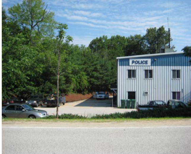
Existing Police Department at Safety Complex
