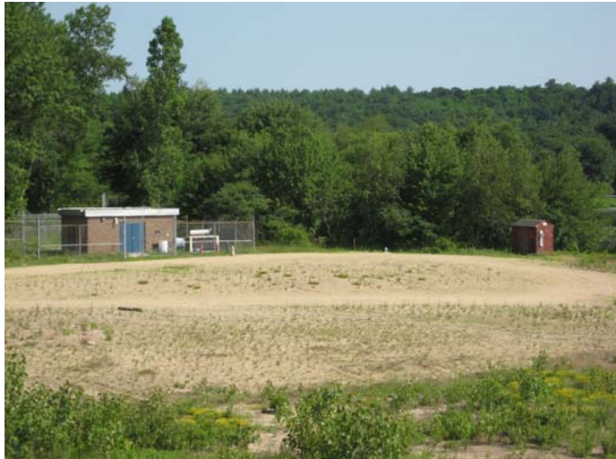
Raymond Well (PW- 1) and Pump House
