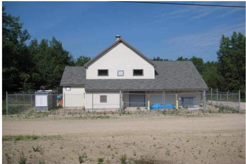
Existing Water Treatment Plant
