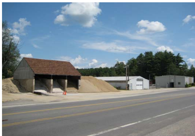
Town Salt Storage Shed
