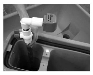
**Step 2**Attach the 150 psi hose with shutoff valve (provided) to the PVC elbow, use teflon tape on all threaded fittings.
