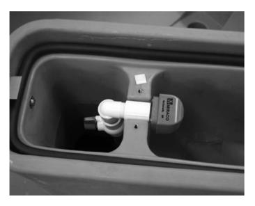
**Step 3**Set the entire assembly into the valve cradle.
