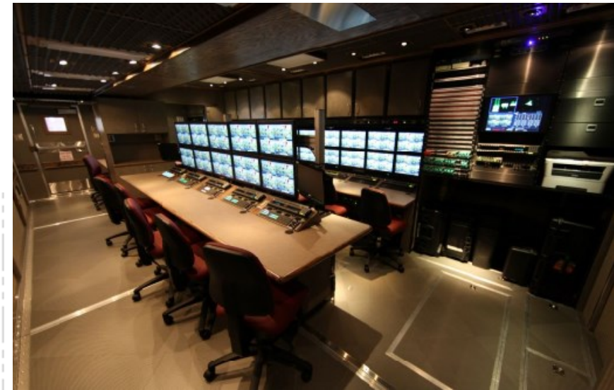
B UNIT WORK SPACE
