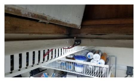
I left the wall switch there, and just wired the Normally Closed (NC) contacts [light turns OFF as switch is pressed by hatch] of the microswitch to those terminals. The microswitch would override the OFF position of the wall switch, but turning on the wall switch would force the light to be always on.
