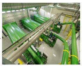
With PWC 2.0 there is no human contact after a waste bag is deposited into a disposal inlet until it reaches its final recycling or disposal destination. Waste workers are completely safe.
