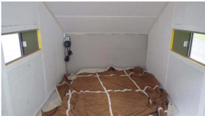
I started with a 4x8 trailer from Harbor Freight and shortened it 18 inches and added a plywood floor. I constructed the walls and framing from 3/4 x 1-1/2 pine and 1/4" underlayment. Everything was glued and screwed together. 3/4" thick foam sheets were glued to the inside walls for insulation.
