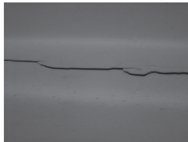
Figure 1: Axial crack in CPVC sprinkler pipe to due preservative oil washed in with the water 100x
