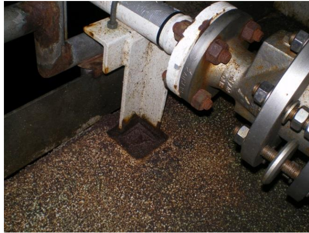
Fig 4 - rusting carbon bolts in stainless substrate
