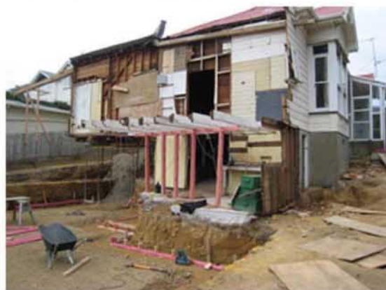
Demolition started 4th April 2010
