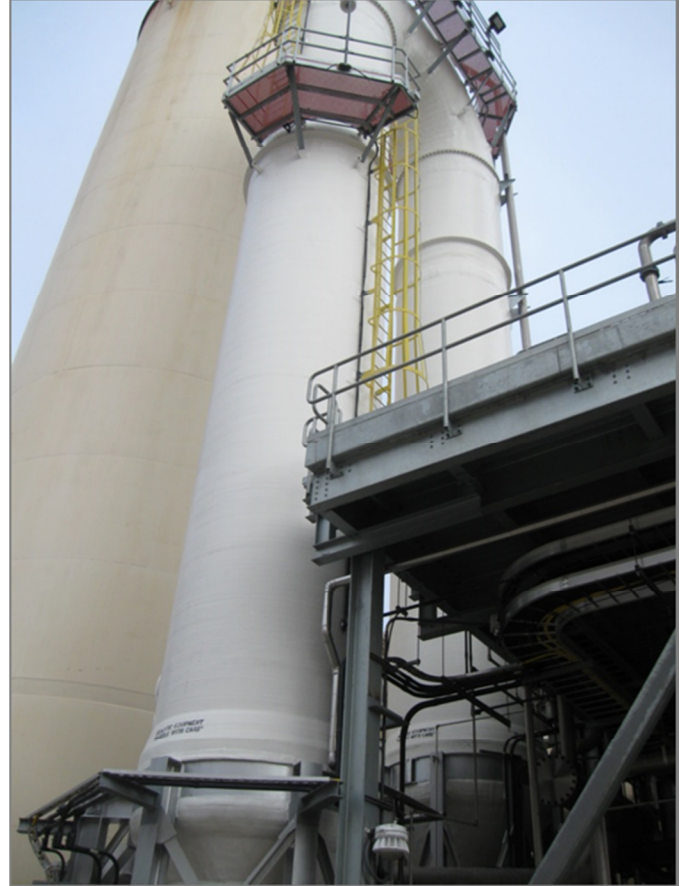
Fig. 2: New Bleach Plant. Final bleached pulp is moved to D2 storage tower prior to entering the pulp machine.
