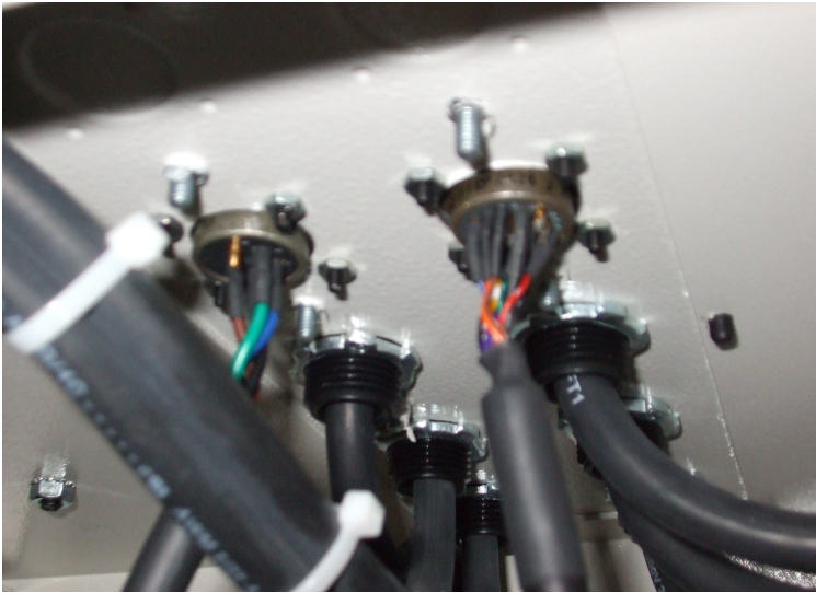
Figure 2. Mount the signal and power wires. If the electrical cabinet already has knock outs, use those holes. Otherwise, a 7/8" (22mm) hole will need to be drilled to allow the cables to enter the cabinet. Important, do not let the cables twist or pull on the wires, they will break with too much force or twist.
