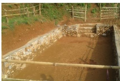
Runoff diversion wall (above), recharge trench and pond (below)
