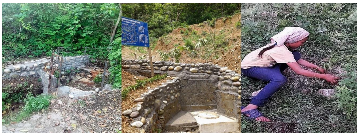
Photo 4 Simple methods to reduce disaster risk at intake, photos by Syangja D-WASH Unit
