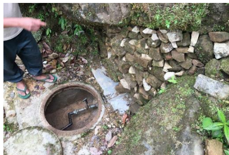
Closed intake with clean fitting chamber.
