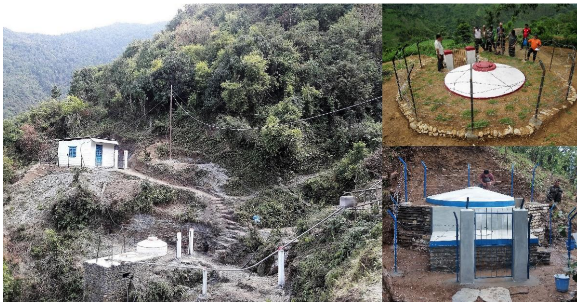
Photo 5: Electric lift and gravity scheme structures, photos by Baglung and Gulmi D-WASH Units
