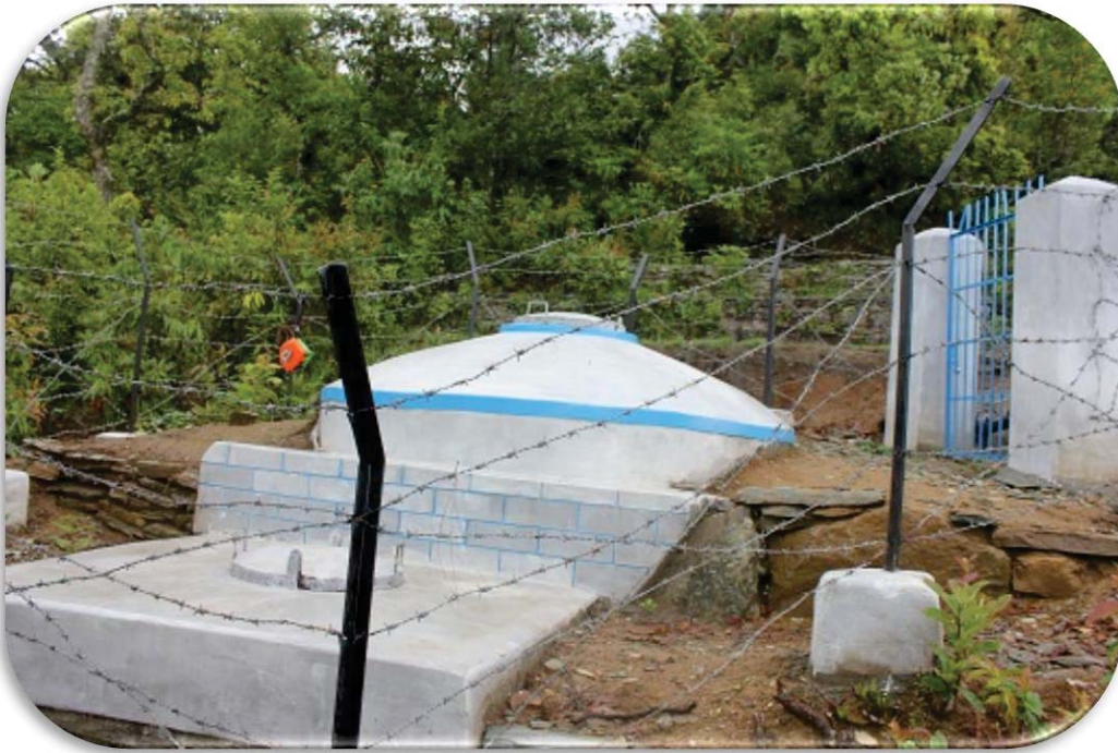
5 M 3 Ferro cement RVT of Chaurasi Dhara DWSS, Dhairing - 7
