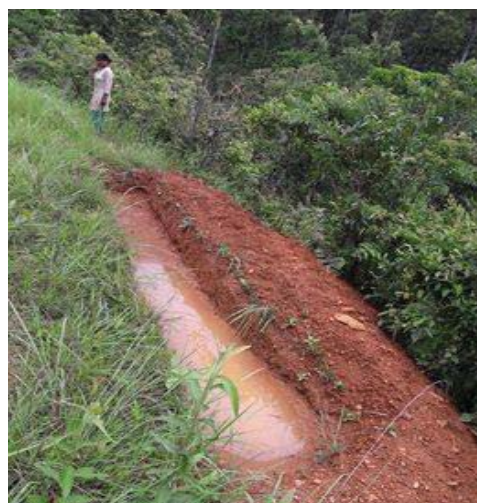
Recharge Trench for spring Revival at Dhamilikuwa DWSS, Ghansikuwa VDC,
