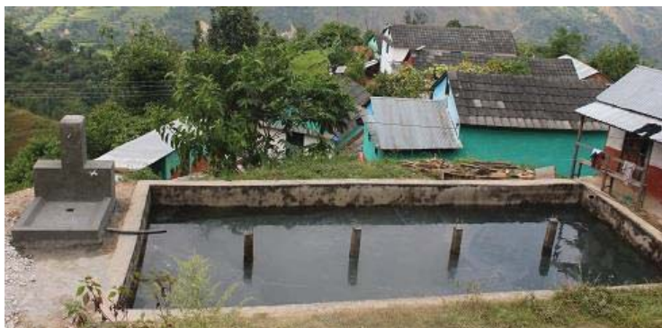
Waste and excess water fed to existing empty irrigation tank through public tap of Kattike Gaihre Asi Mure DWSS, Barrachaur-7 Photographed on 13.10.2015
