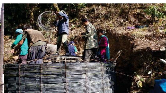
Construction going on RVT of chhelderkhola DWS
