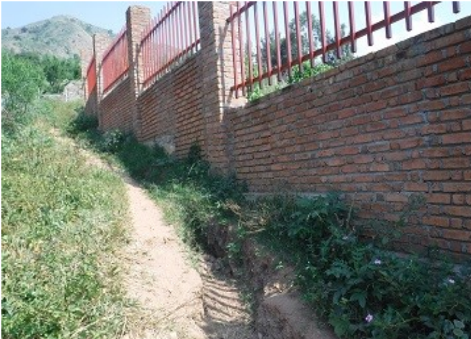
We are so thankful the security wall at CCC is finished!
