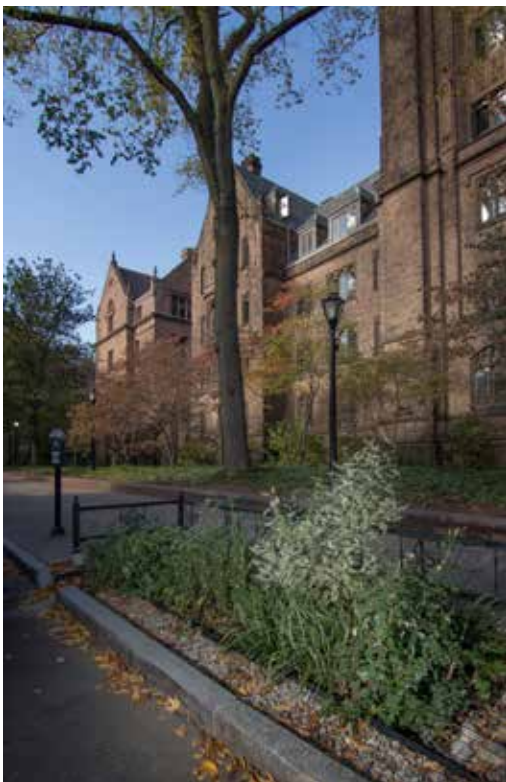
More than 30 bioswales that appear as miniature urban rain gardens were created by the City of New Haven to capture rainwater runoff and prevent flooding caused by heavy downpours and overtaxed storm drains. The city plans to install up to 300 more, 200 in the downtown area.
