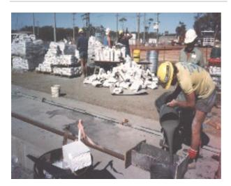
A high-strength free flowing cementitious grout based on non-reactive aggregate. Low alkaline shrinkage compensated Portland Cements with selected admixtures produce a chloride free grout, containing non-corrosive metallic additives. TamCrete HF contains a maximum size aggregate of 2mm and is suitable for grouting thicknesses of between 5mm and 75mm.
