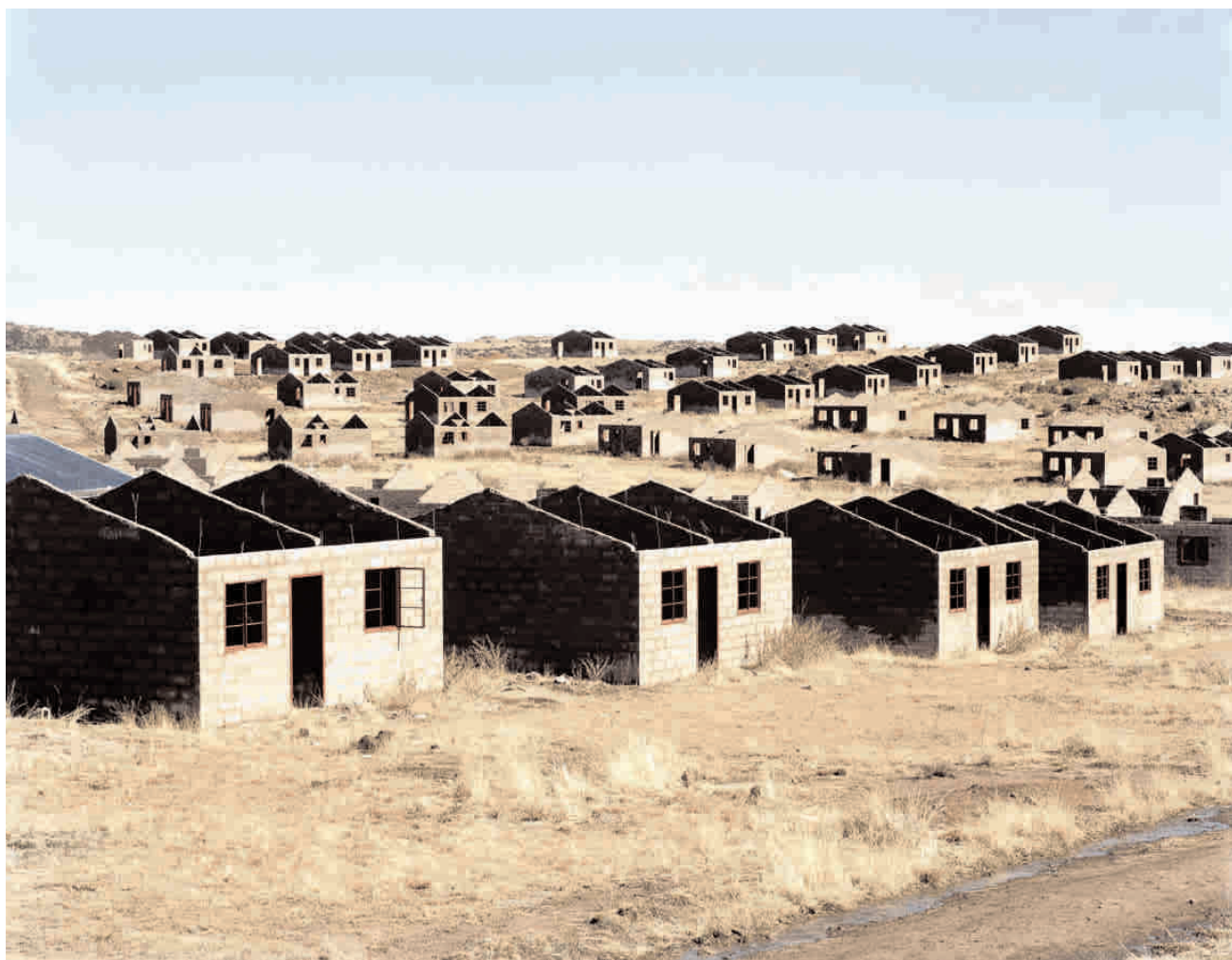
Stalled municipal housing scheme, Kwezinaledi, Lady Grey, Eastern Cape. 5 August 2006. David Goldblatt's photography has always been politicised. Corruption and inefficiency are some of the issues that his work explores
