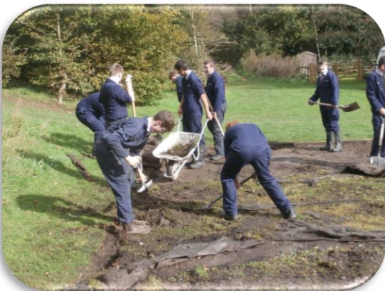
Construction Pupils creating an outdoor learning environment
