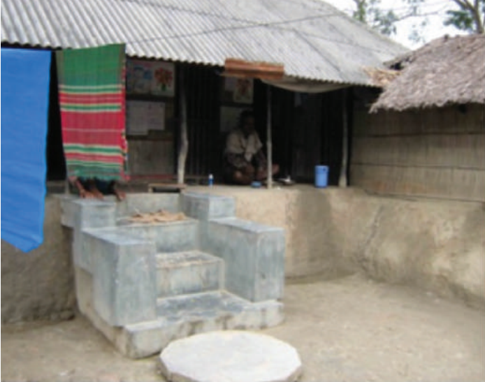
Low drooping eaves of roof area designed to reduce uplift during storm. Existing verandah provides room for household activities
