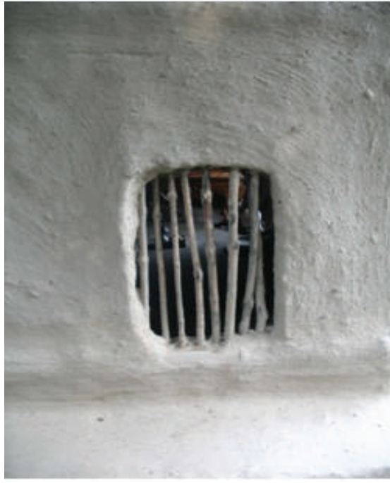
Window made of local Goran wood embedded in mud wall
