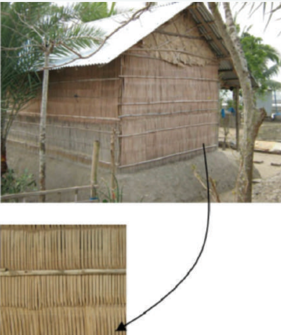
Traditional wall made of treated nipa palm tree, on high raised mud plinth
