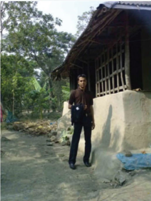
Raised plinth to protect from flood water
