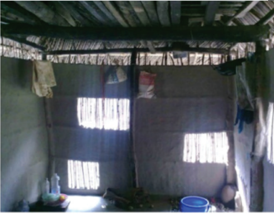
Windows at various levels for maximizing cross ventilation
