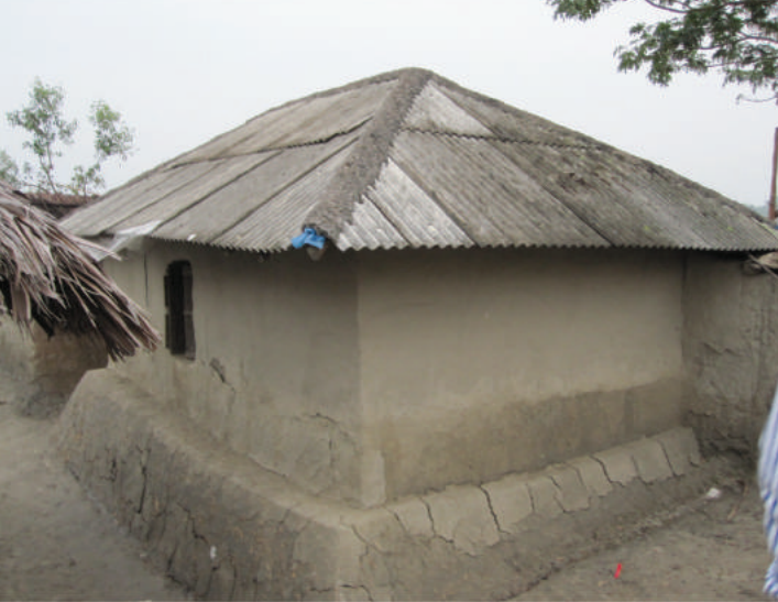
Use of asbestos roof in existing house hold has been seen, which is carcinogenic and compromises health safety issues, and example of mud plinth wall erosion
