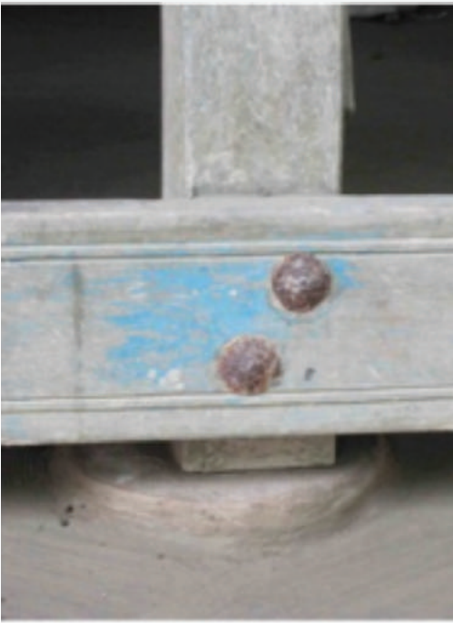
Protection of wooden pillar base & attachment to mud plinth
