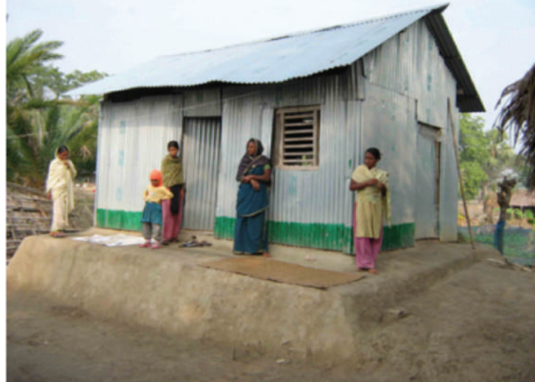
Example of typical house made by NGO, Absence of verandah, C.I sheet walls & pitch roof is vulnerable and poses risk during storm
