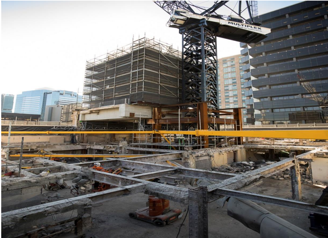
Shell House – Demolition
