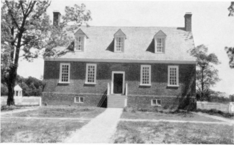
WARREN HOUSE AT SMITH FORT
