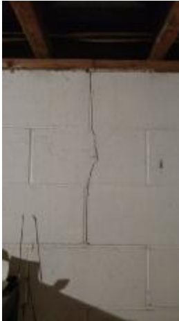
Settlement crack
