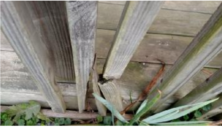
Broken baluster
