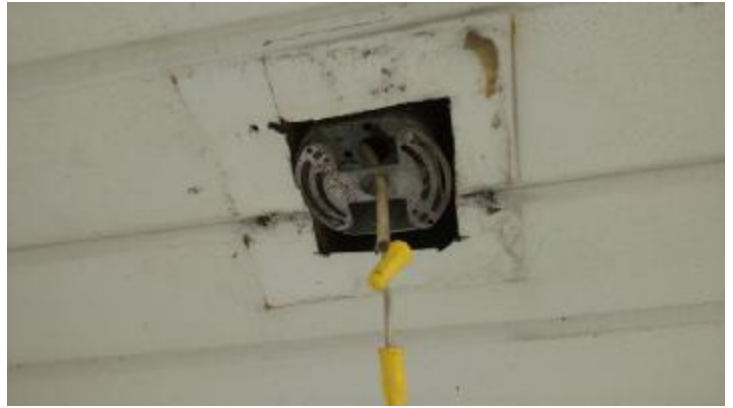
Exposed wires
