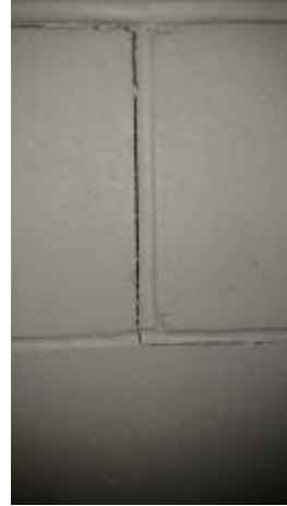
Settlement crack
