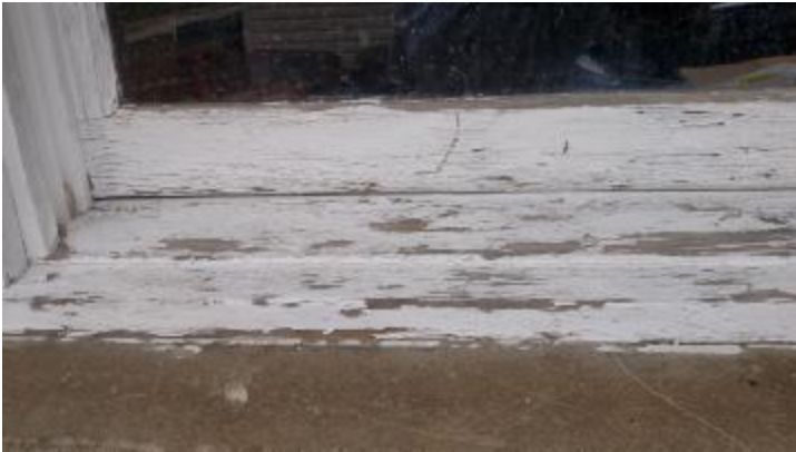
Paint window trim
