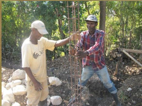
Pastor Roland (right) helps with the construction work at Dos Palais.
