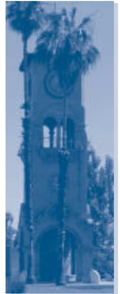
The Kern County Museum's tower makes this facility hard to miss.
