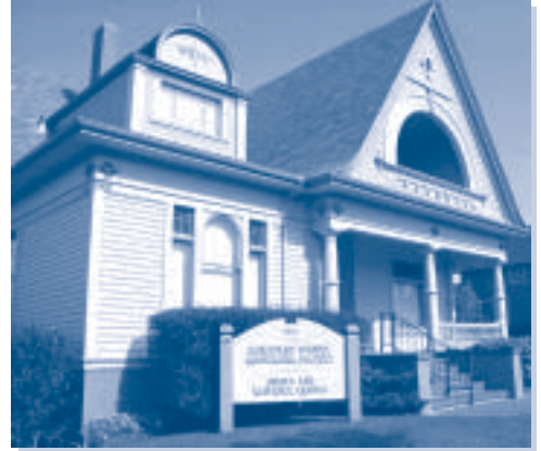
The Humboldt County Historical Society's lovely headquarters building
