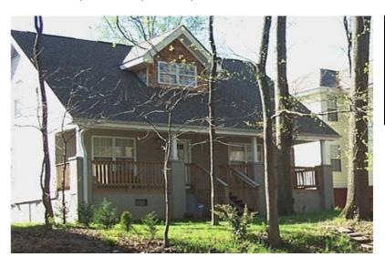
**Non-Visitable Home:** Steps at this home prevents accessible entry. With steep terrain, a zero-step entry can be located at back of the home.
