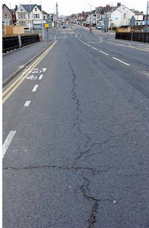
Crack in railway bridge in Blackpool
