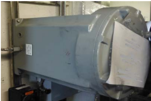
Figure 2: Example of Explosion-Proof Enclosure
