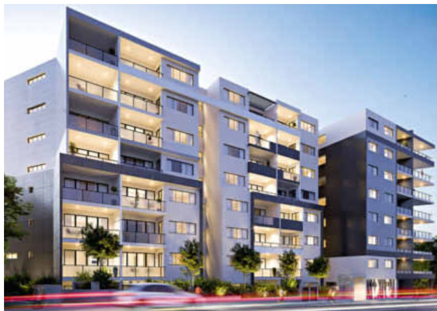
Jacinta Burwood has 87 apartments of various sizes in a seven-storey building.
