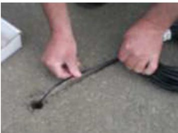
Cut a 5mm slot in tarmac road surface for the cable. Cut a trench for a duct in gravel or hardcore. Lower in the sensor until the yellow top is 8" below surface. Pour kiln dried sand in to fill the hole up to the top of the sensor. Fill the last 8" with a more structural plug of post mix or cold black top.
