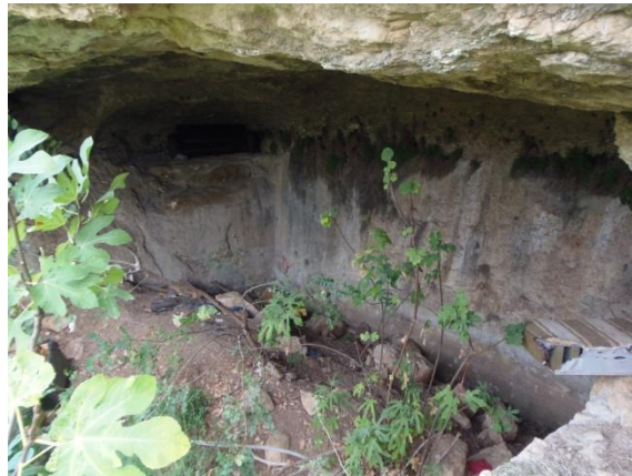
Figure 7 Cistern overlooking the monastery.
