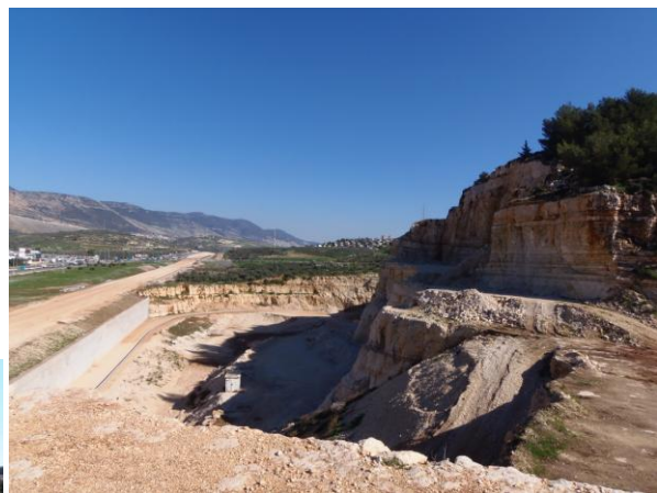
Figure 35 The north side of Horvat Midrasa was quarried in the 1930s, and has now been further cut away for the Karmiel-Acco railway.
