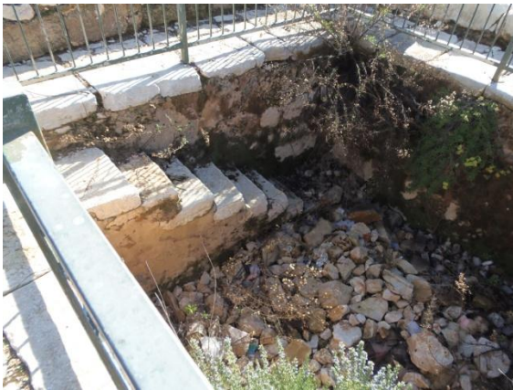
Figure 22 The wine collecting pit, with access stairs.
