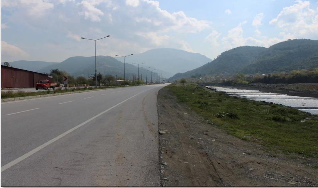
Fig.4. The roadside verge and adjacent stream bank zone in the study plot.
