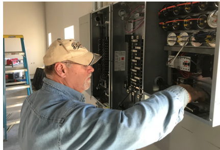
Toby Roberts installed the 3 phase rotary phase converter and electrical panels.
