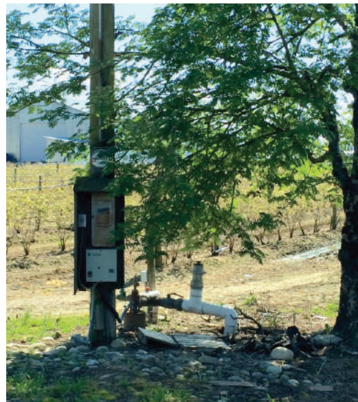
Photo 2. Well too close to power pole
