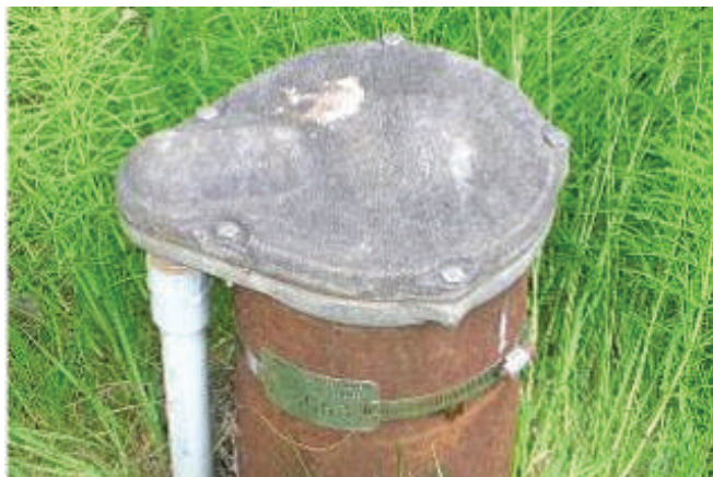
Photo 5. Aluminium well cap on a domestic well
