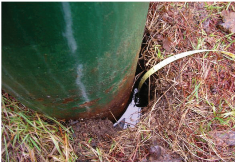
Photo 1. Visible void space around well
