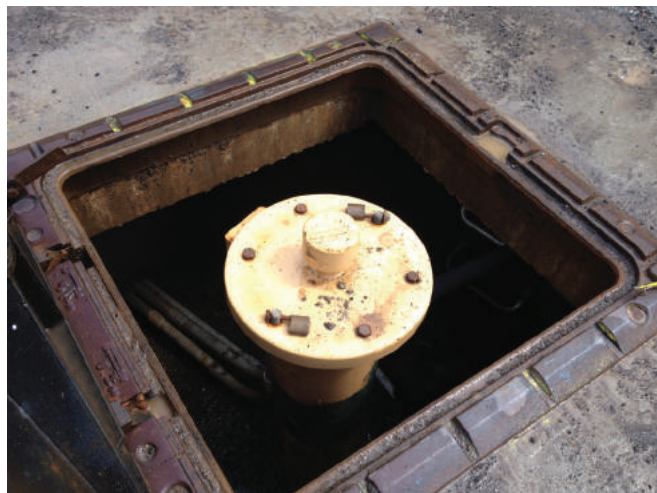
Photo 3. Example of a well in pit
