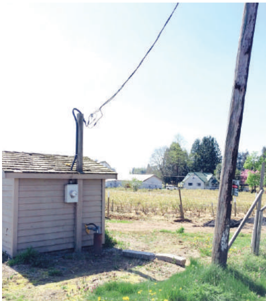
Photo 1. Pump house with power line obstruction
