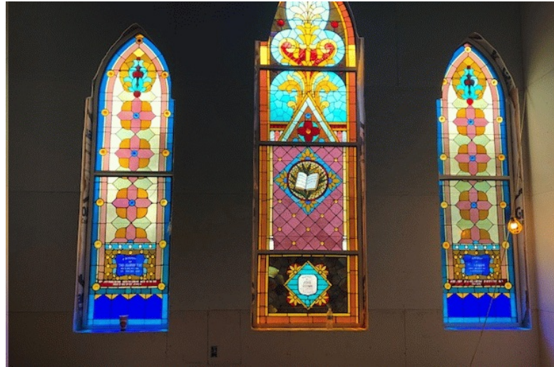
Windows in Choir Room Drywall has been hung.
