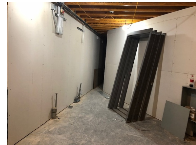
Door thresholds stored in area behind the stage.
