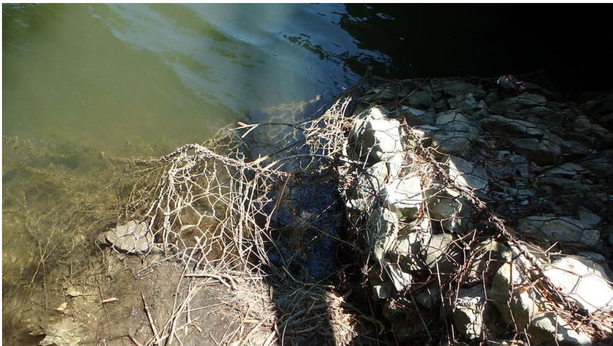
Figure 16 Deteriorated Gabion Basket
