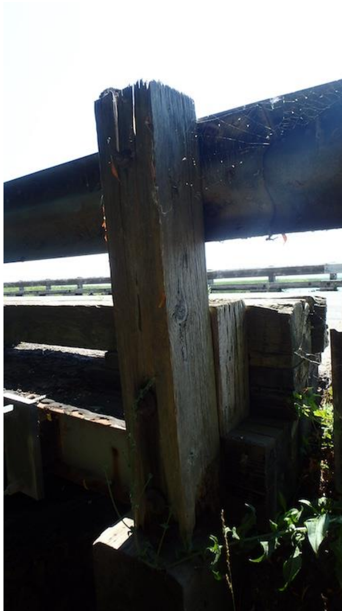
Figure 21 Typical Post Deterioration
