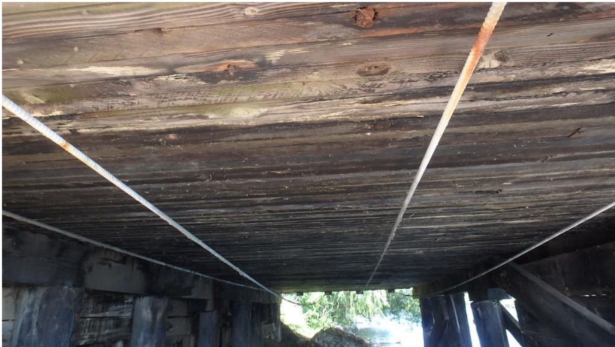
Figure 15 Loose Post Tension Strands
