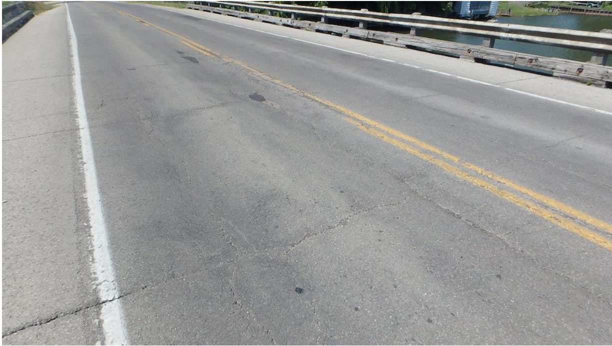
Figure 28 Transverse Cracks and Settlement on Deck Wearing Surface
