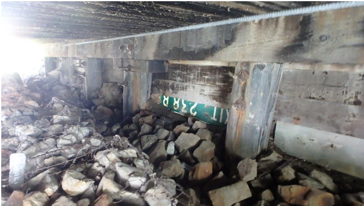
Figure 13 South Abutment Deterioration
