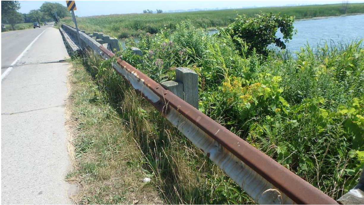
Figure 24 Corrosion on Guiderail
