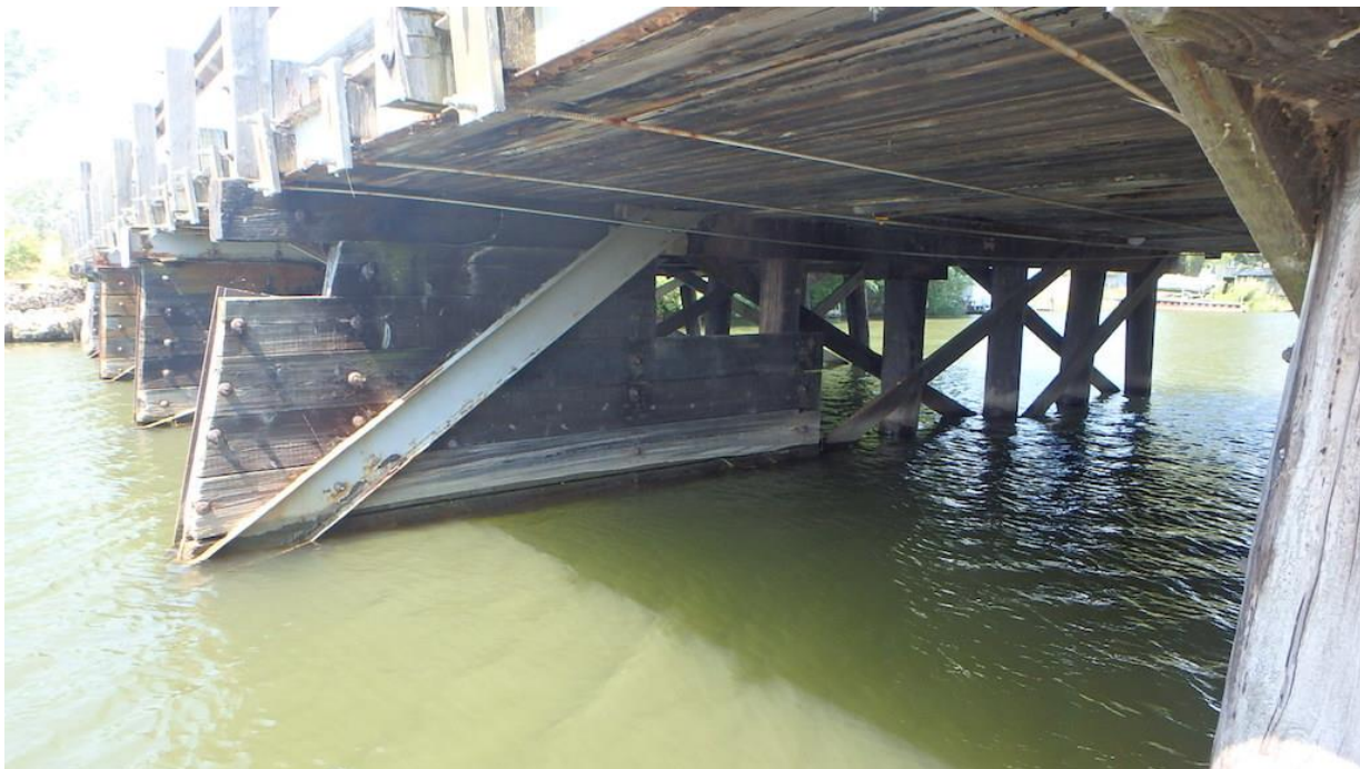
Figure 14 Steel Pier Reinforcement
