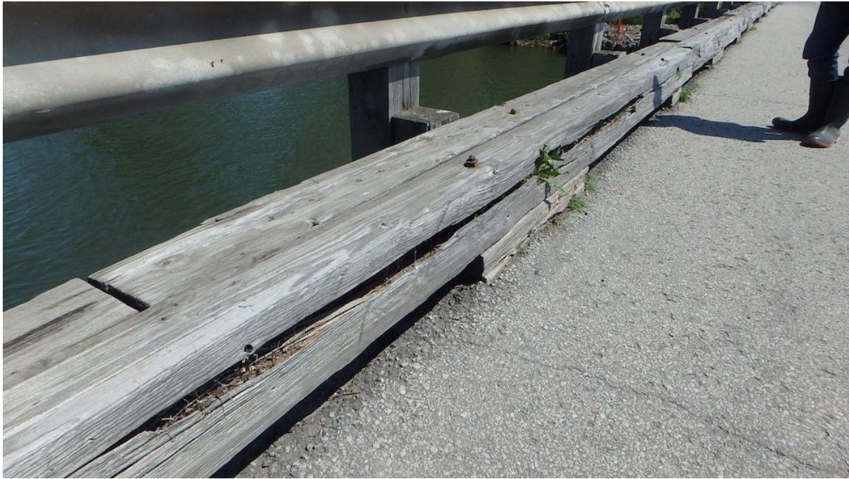
Figure 22 Deterioration of Wood Curb
