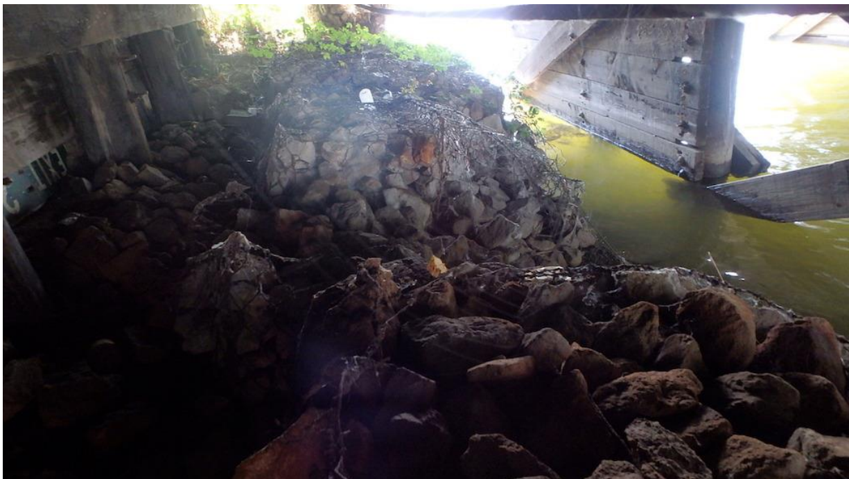
Figure 18 South Gabion Wall Deterioration
