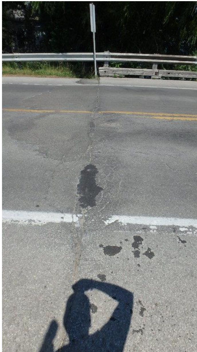
Figure 26 Settlement at North Joint
