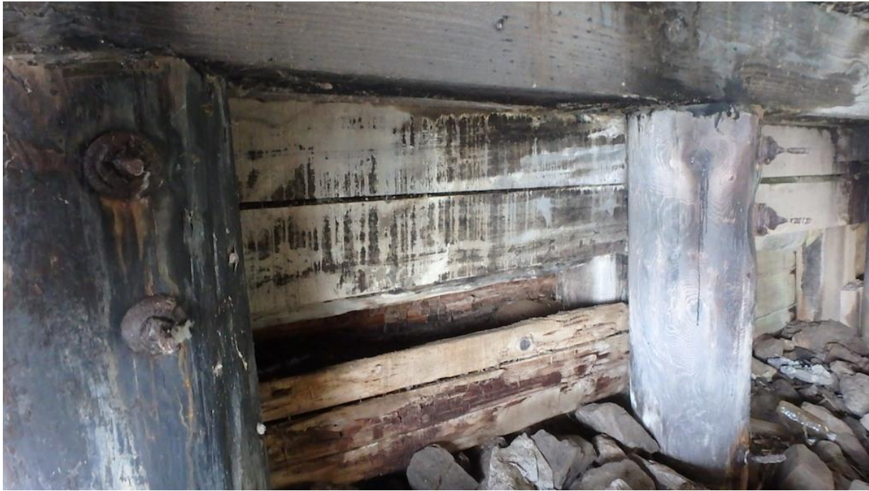
Figure 17 Missing Board in Ballast Wall
