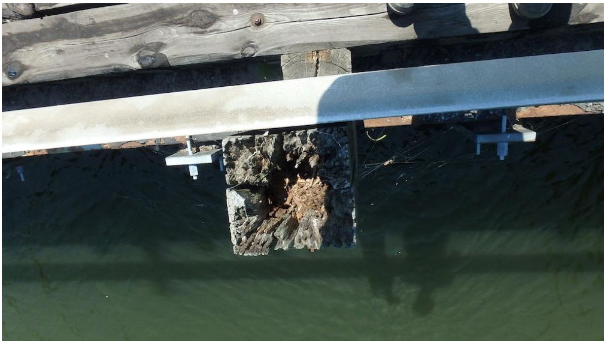
Figure 23 Insect Damage to Guiderail Post
