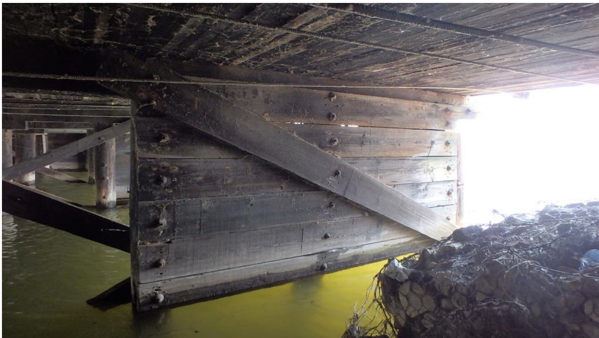
Figure 12 Shear Panel
