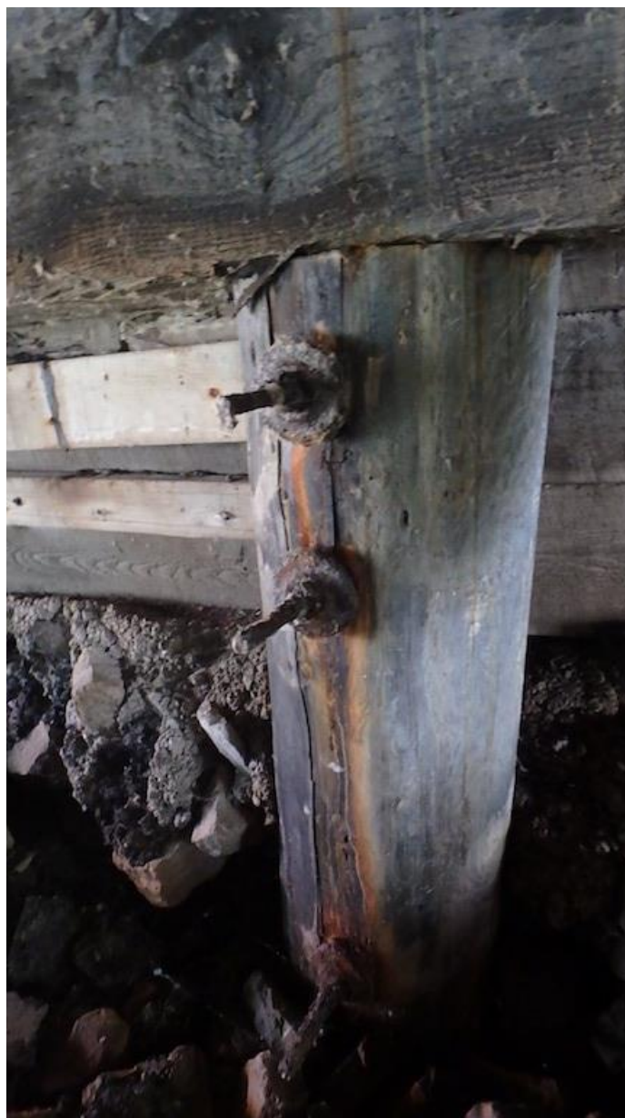
Figure 19 Typical Wood Pile
