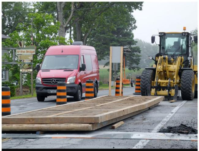
Rig mat decking has been placed on the causeway between Long Point and Port Rowan as a temporary repair for a wooden bridge that is beginning to fail. **MONTE SONNENBERG / SIMCOE REFORMER**
