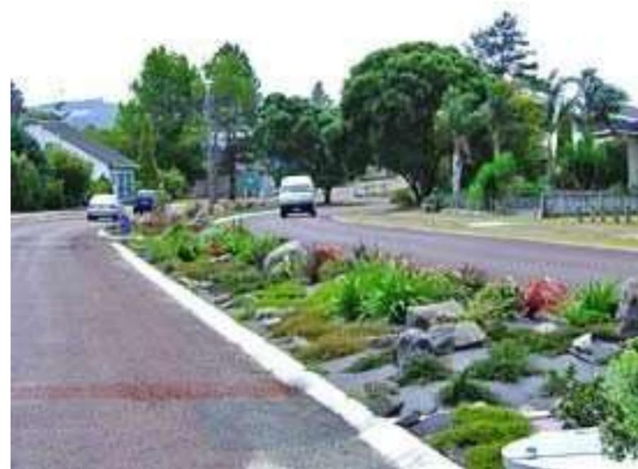
This system was installed in Pauanui, a coastal community, in 2009. It distributes tertiary treated waste using a subsurface drip system over a combination of parks, planted road median strips and a grassed air field. Located on a thin spit of sand, the area's population fluctuates due to holiday visitors. As some of its drinking water supply is drawn from shallow bores, the system had to be carefully designed to prevent contamination.
