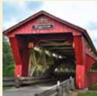
Length: 102 feet Year: 1873 Builder: Partridge Spans: Little Darby Creek Historical Marker
