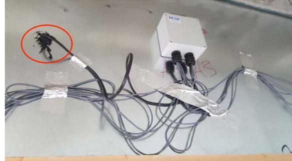
Figure 13. Differential pressure sensor installation
