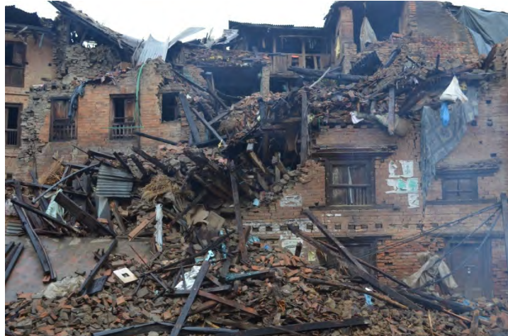
The 2015 Gorkha Earthquake damage in Bhaktapur city.
